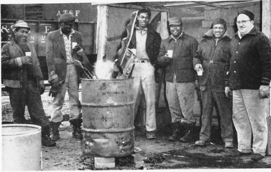
Freight Handlers (left to right) Pat Cornish, Richard Knight, Mat Paris, Willie Davis and Harry Guy, plus Gerald Ricciardi of Millwrights made up the crew which had been loading and unloading material in the city's freight yard since the washout of the Dublin St. wooden trestle in the August flood.
